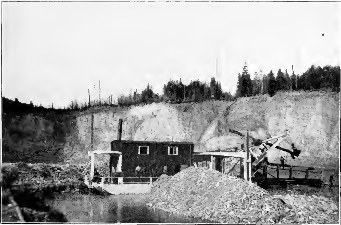
NEWALL DREDGE—CUTTING THROUGH BAR—FRASER RIVER.
